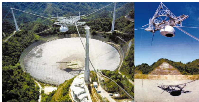
Figure 1. SETI@home uses the National Astronomy and Ionospheric Center's 305 meter telescope at Arecibo, Puerto Rico. The inset at right shows the details of the "carriage house" structure. The SETI feed is the vertical structure extending downward from the carriage house. (Photos courtesy of NAIC—Arecibo Observatory, a facility of the NSF. Photos by David Parker and Tony Acevedo.)
